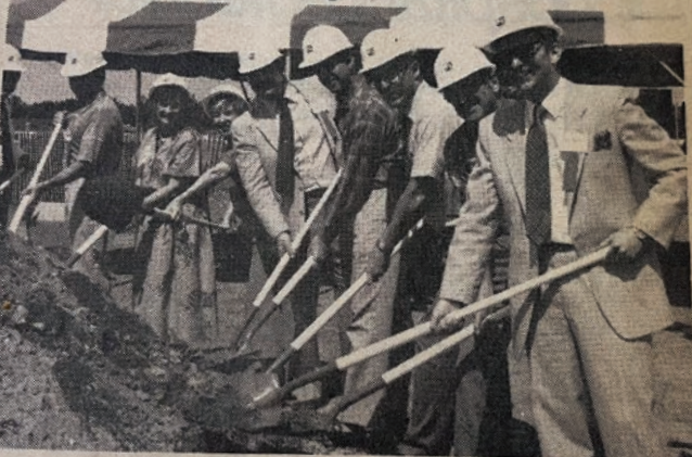
Knollwood Place, rental apartments for senior adults, held groundbreaking ceremonies May 31 at its location on the Jewish community campus in St. Louis Park. The project is owned and developed by Community Housing and Service Corporation. Shown above are the CHSC past presidents, along with executive director Jon Weiss and current president Allan Swartz. Left to right are Mel Goldfein, Bernie Herman, Arline Bloom, Sandra Freidman, Weiss, Ben Steinberg, Ray Harris, Harvey Ratner and Swartz.
